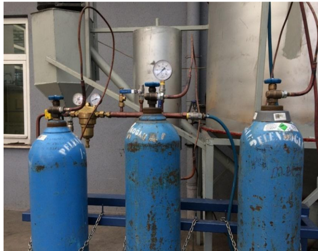
Figure 6. Argon gas system.
